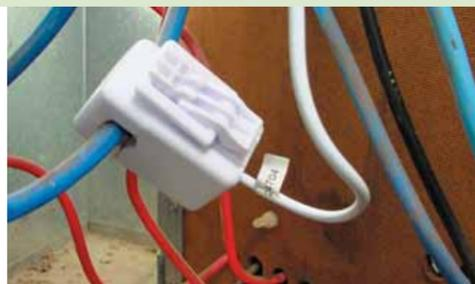
1 The Clip-On Sensor simply attaches to the main active or phase cable at the switchboard.
